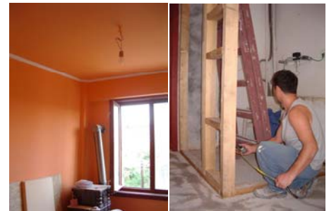
The renovation has started
