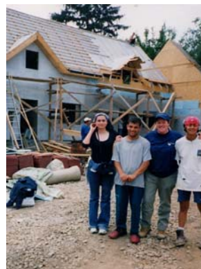
At HFH Cluj site
