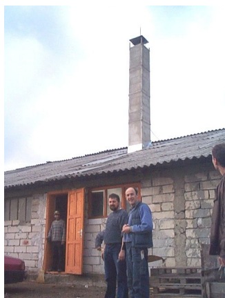
The new chimney of the Carpentry shop
